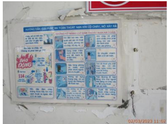
60. Fire escaping instruction in case of fire emergency.jpg
