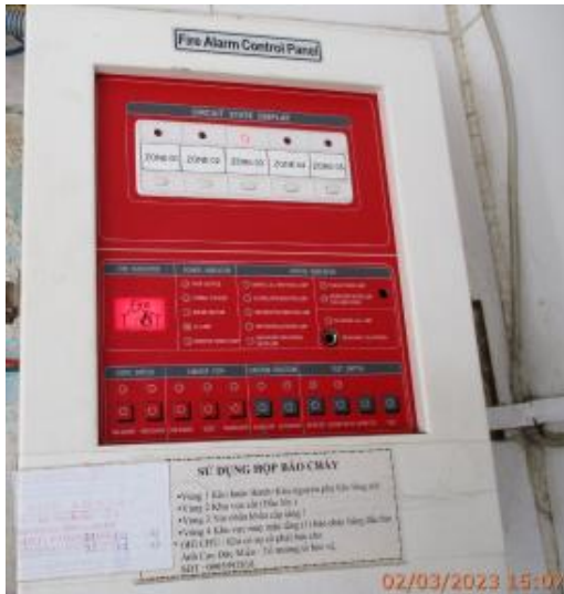
21. Fire alarm control panel testing onsite.jpg
