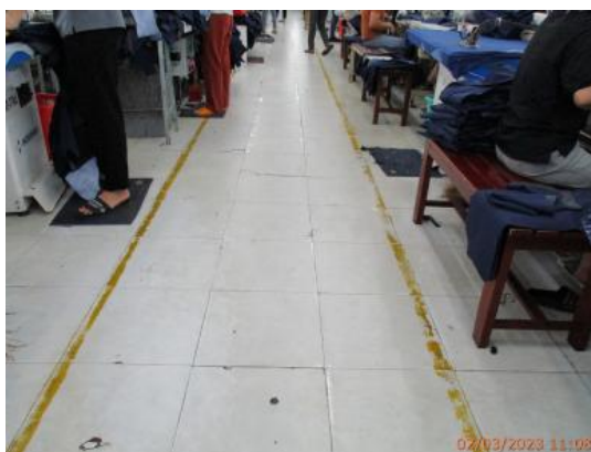
83. Finding - The evacuation marking was fade on floor of the sewing area.jpg
