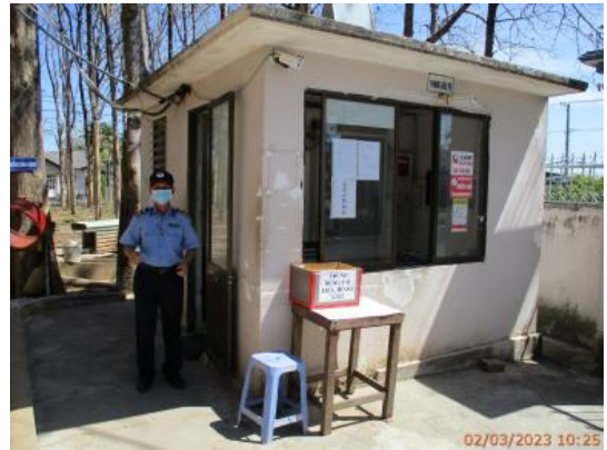
4. Security room at main gate.jpg
