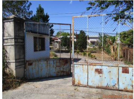
74. Dormitory for employee - entrance.jpg
