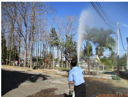
35. Fire hose testing onsite.jpg
